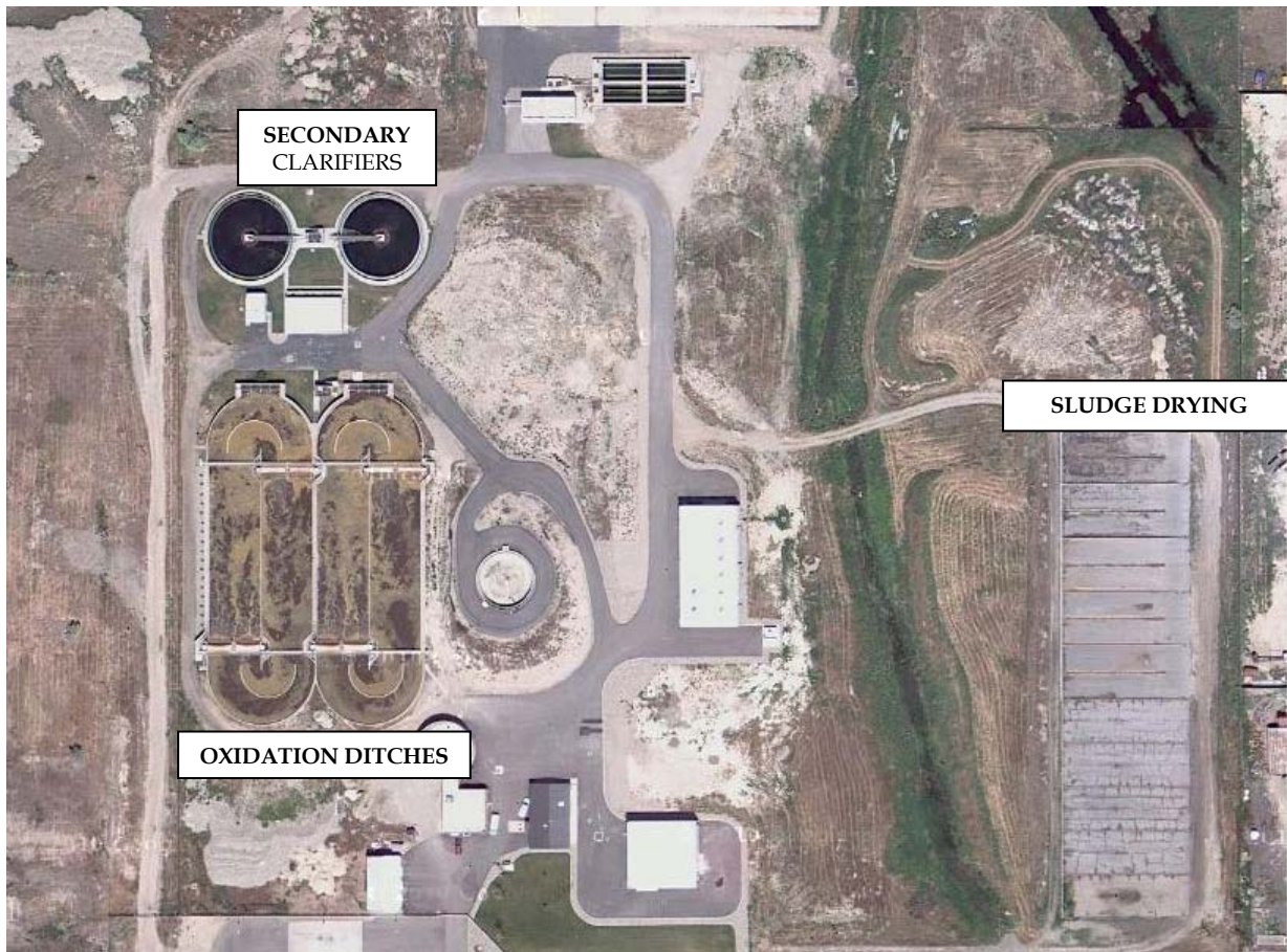
FIGURE 2 Aerial View of the Facility
